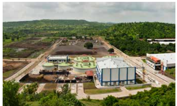
Pilot Plant for Bio-Gas & Green Energy
