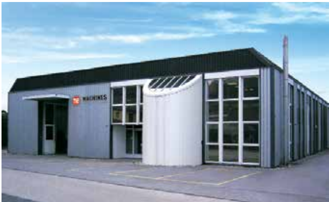
Driptube and Pipe Manufacturing Equipment: THE Machine S.A. (Switzerland)
