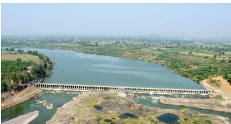
Kantai Bandhara, with water backed till 9.5 kilometers, and a capacity of 200 crore (approx) liters was constructed by Jain Irrigation at a cost of Rs. 7.86 crores. The water will be shared equally by surrounding eight villages and Jain Irrigation.
