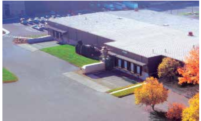
Plastic Building Products: Nucedar Mills Inc., Chicopee (USA)
