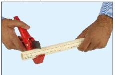
It is important to cut the pipe square by using suitable pipe cutter. A square cut pipe provides the surface of the pipe with the maximum bonding area. Tools used to cut pipe must be designed for plastic use and must be in good condition. If there is any indication of pipe damage or evidence of pipe cracking, cut off at least 50mm beyond any such defect.
