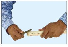
A chamfering tool or a file is suitable for this purpose. A slight bevel (approximately 10°-15° chamfer and a minimum width of 3/32 of an inch) shall be placed at the end of the pipe for ease entry of the pipe into the fitting socket. This will minimize the chance that the edges of the pipe will wipe solvent cement or will scrape softened surface material from the fitting socket during the insertion of the pipe.
