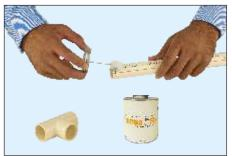
Apply Permafix CPVC solvent cement to the pipe end. Be aggressive to break down the surface tension and to soften the surfaces.
