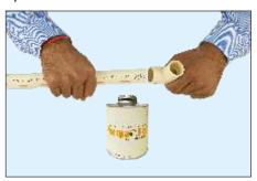
Hold the pipe and fitting together for approximately 30 seconds to avoid push out. Adjust the hold on time based on surrounding conditions.
