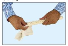
Using a clean dry cloth, wipe any dirt and moisture from the fitting socket and the pipe end. Moisture will slow the cure time, and excessive water can reduce joint strength.
