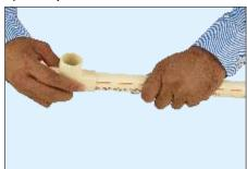
The pipe should enter the fitting socket easily 1/3 to 2/3 of the socket length for a tight interference fit. Contact between pipe and fitting is essential in making a good joint. This contact allows the solvent cement to effectively join the pipe and fitting.
