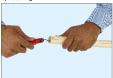
Burrs and filings can prevent proper contact between pipe and fitting during assembly, and must be removed from the outside and the inside of the pipe before assembly. Use de burring tool to remove such burrs.
