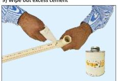
A bead of solvent cement must be around the entire socket fitting entrance. With a clean, dry cloth, remove the excess solvent cement from the pipe and fitting socket entrance. This will allow the solvent to evaporate from within the joint.
