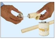
Apply a very light layer of solvent cement to the inside of the fitting socket. This will prevent puddling of the solvent cement inside of the pipe or fitting. Excessive solvent cement applied to the fitting socket can cause the joint to clog and the wall of the pipe or fitting to weaken due to softening by the accumulation of the excessive solvents.
